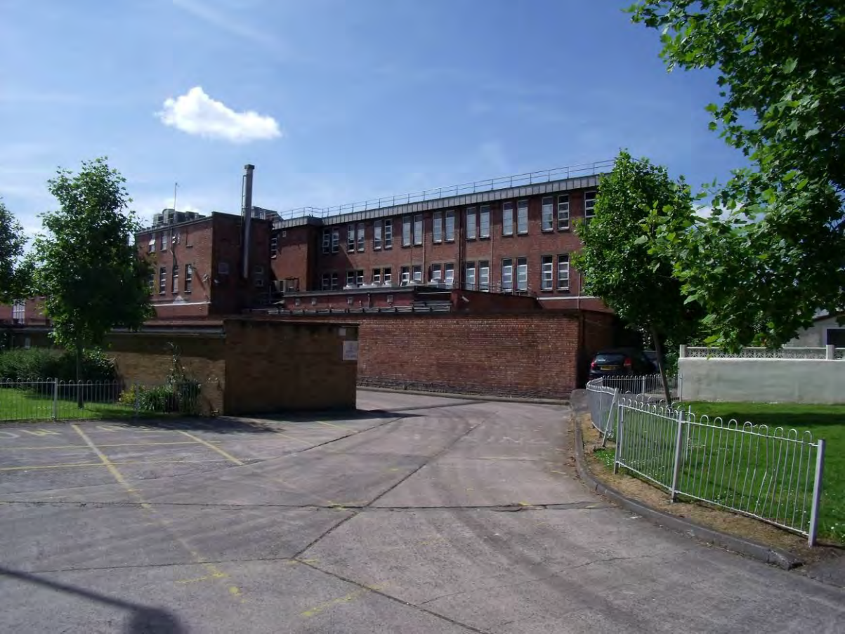
View of rear of site from access to garage block adjacent to Littlecross House
